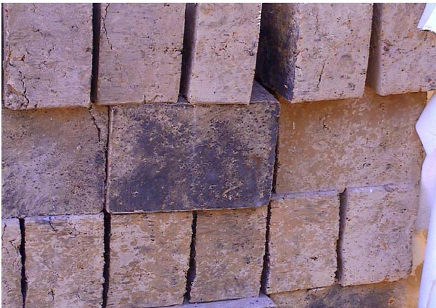
**Figure 1 - Whittlesea Mud Bricks Out in the Weather 17/03/05**
