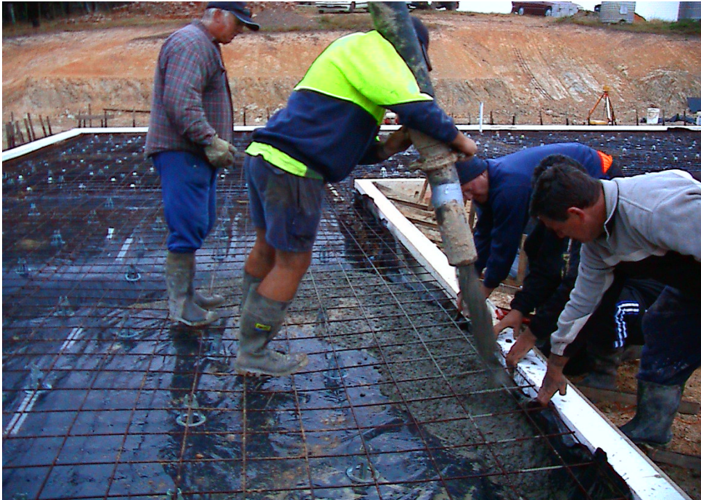
Figure 2 - Pouring at 100+ Slump
