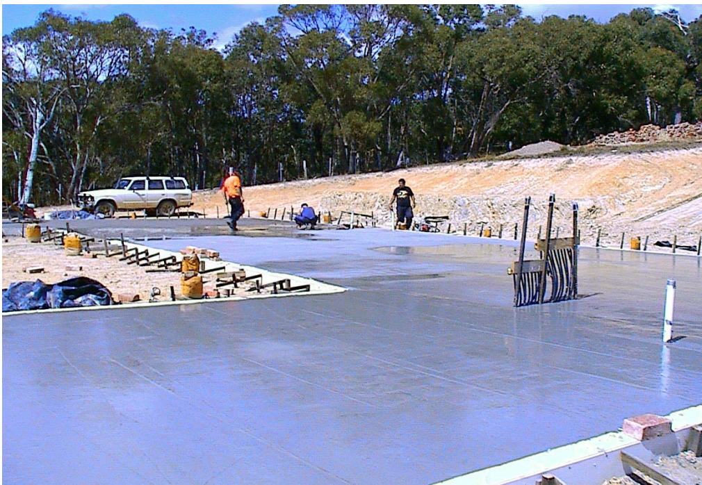
Figure 3 - The Slab Drying Off (It rained!)
