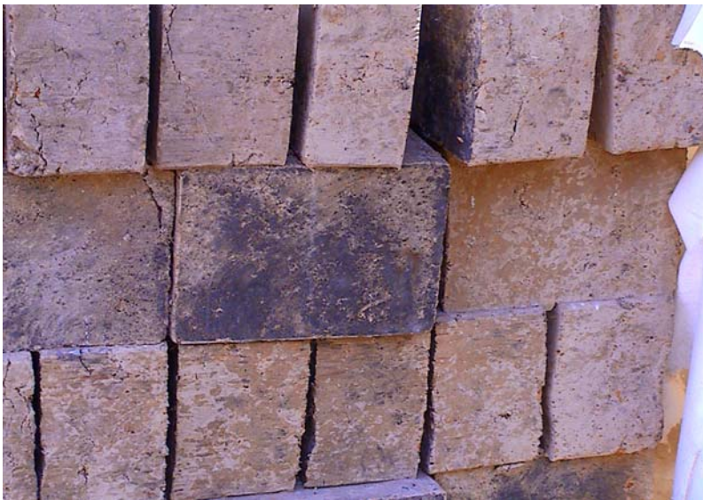
Figure 1 - Whittlesea Mud Bricks Out in the Weather 17/03/05
