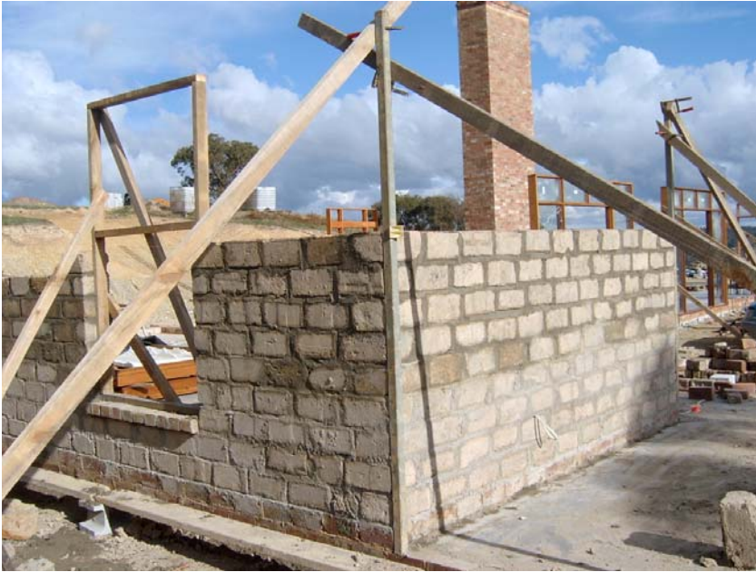
Figure 3 - Detail of Corner Watson Whittlesea Project Home 15/08/05
