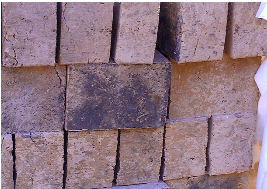
Figure 1 - Whittlesea Mud Bricks Out in the Weather 17/03/05
