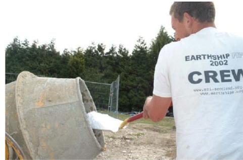
We have mainly been using the 1 OPC, 2 MgO, 9 Ballast mix as a mortar for bottle walls and other minor works. It was a pleasing mix to work with, stiff yet pliable and workable.
