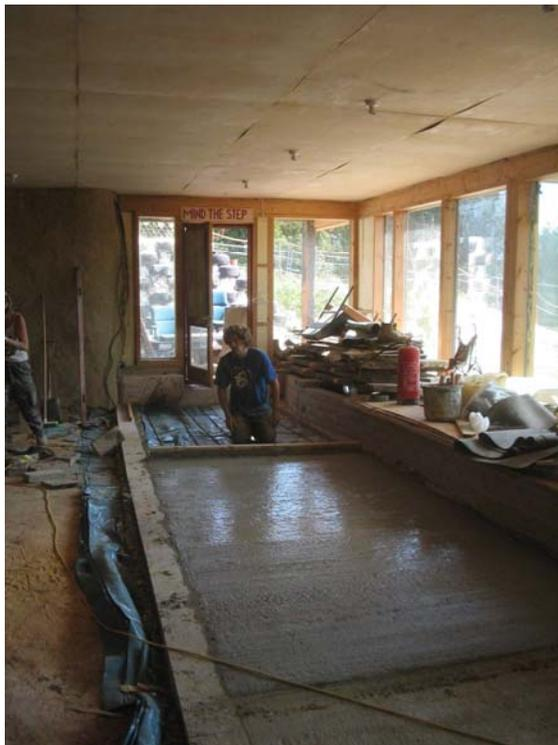
As the eco-cement 28 day test gave a compressive strength of 19.6 N/mm<sup>2</sup> for 1 OPC, 2 MgO, 9 Ballast, compared with a PC concrete test block (1-OPC: 3-Ballast) of 36.2 N/mm<sup>2</sup> and was sufficient for structural works, we decided to use eco-cement formulations for our floor slabs from then on. This may have been a risk, but at least a calculated one.
