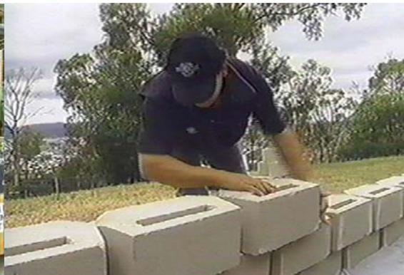
**Figure 4 - Laying Eco-Cement Blocks**
