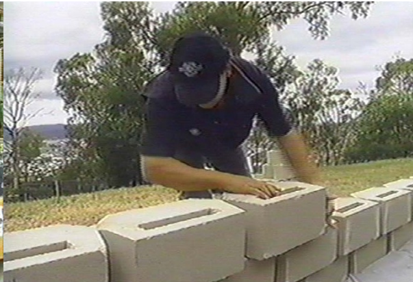
Figure 4 - Laying Eco-Cement Blocks
